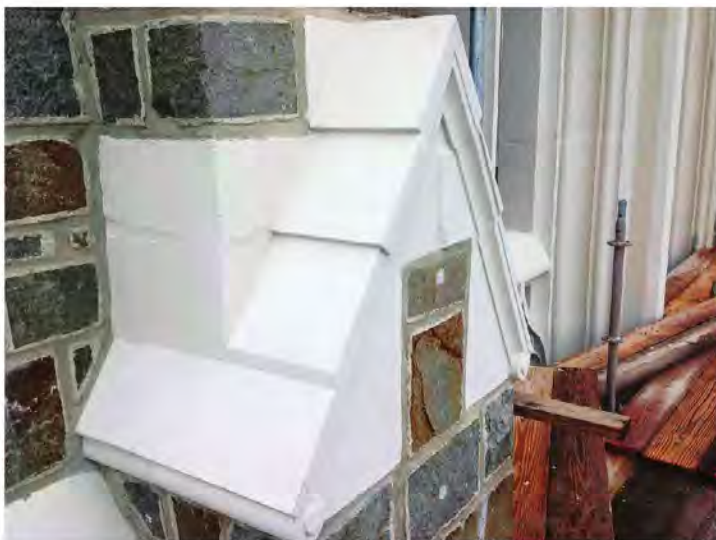
Images before, during, and after repair and coating. Before a coating is applied, the substrate must be restored to a smooth, sound condition.
