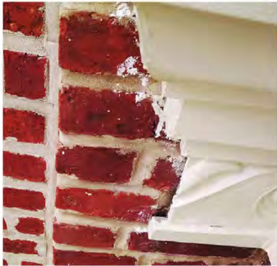
Failure to mask adjacent surfaces during coating application can leave indelible marks.
