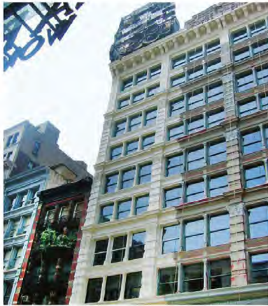
Coating replacement projects can restore historic buildings to their original appearance.
