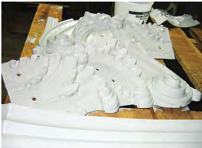
The restoration and recoating of this cast iron element—shown here before and after—required offsite conservation.
