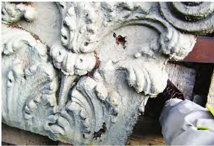
Failure to mask adjacent surfaces during coating application can leave indelible marks.
