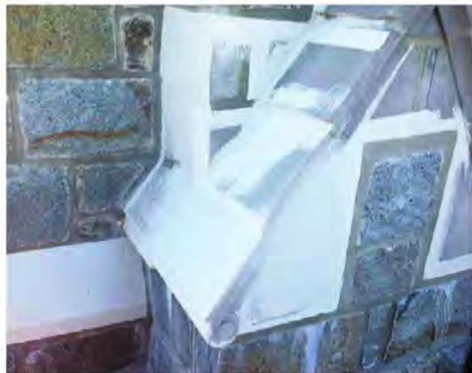
Images before, during, and after repair and coating. Before a coating is applied, the substrate must be restored to a smooth, sound condition.
