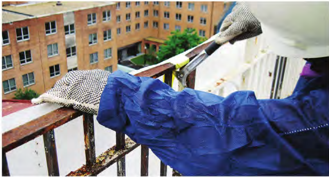
The removal of a failed coating.
