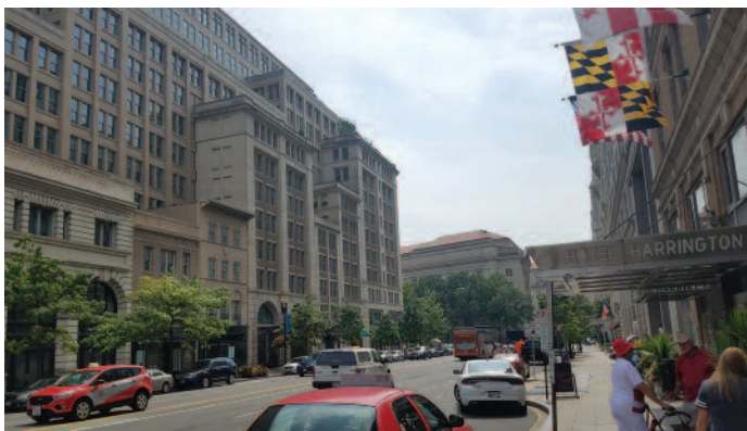
Roof-terrace surveys and replacements at this Washington, D.C., mixed-use development focused on details, from flashings to drainage, that are easy to overlook.
