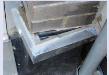
Displaced/damaged flashings.
