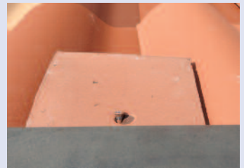
Exposed fasteners.
