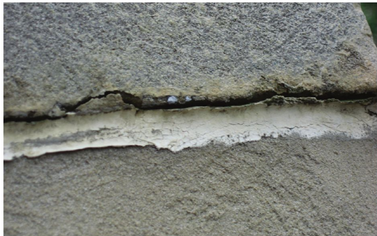
Façade sealant replacement begins with complete removal of existing sealant and backer rod.
