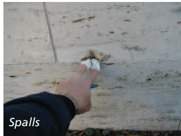
Common problems with thin stone marble facades.
