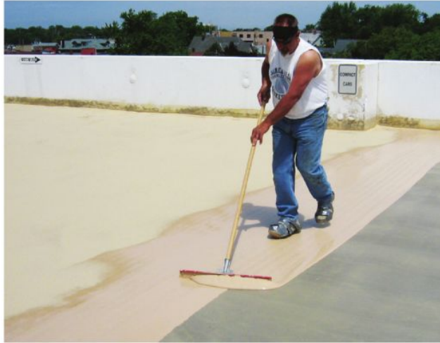
Installation of a traffic-bearing membrane involves multiple steps, including application of a liquid-applied coating (left) and integration of a textured wearing surface (right). The resultant membrane protects against corrosion, but requires maintenance and periodic reapplication.
