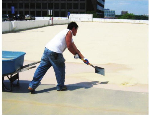
Installation of a traffic-bearing membrane involves multiple steps, including application of a liquid-applied coating (left) and integration of a textured wearing surface (right). The resultant membrane protects against corrosion, but requires maintenance and periodic reapplication.
