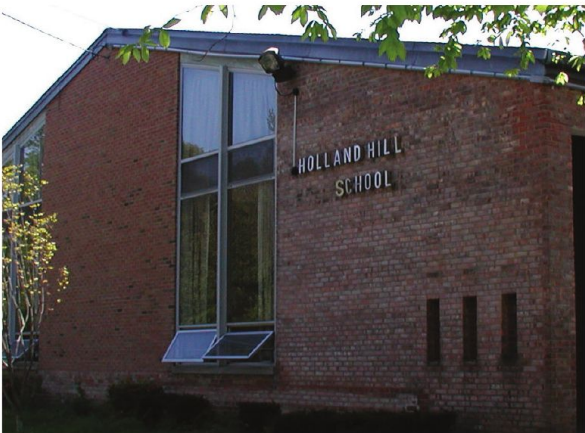
When open, awning windows create a canopy-like projection, offering protection from the elements.
