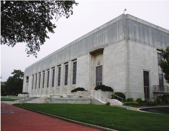
Assessment of the historic windows on this rare book research library involved evaluation of 11 distinct window types for efficiency, waterproofing, and finish integrity.
