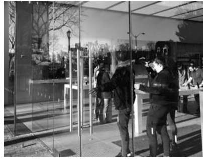
Without weatherstripping, these doors look sleek, but air infiltration may be an issue.
