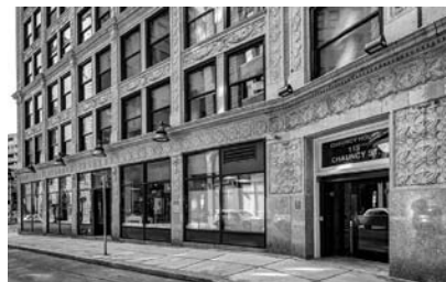
▲ Chauncy House in Boston, Massachusetts. Facade Restoration, Including Storefronts.
