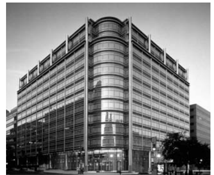
▲ 1900 K Street Office Building in Washington, District of Columbia. Storefront Revolving Door Assessment.
