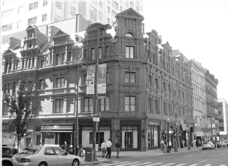
▼ The Goodwin Hotel Hartford, Connecticut. The hotel after Hoffmann Architects' award-winning restoration.
